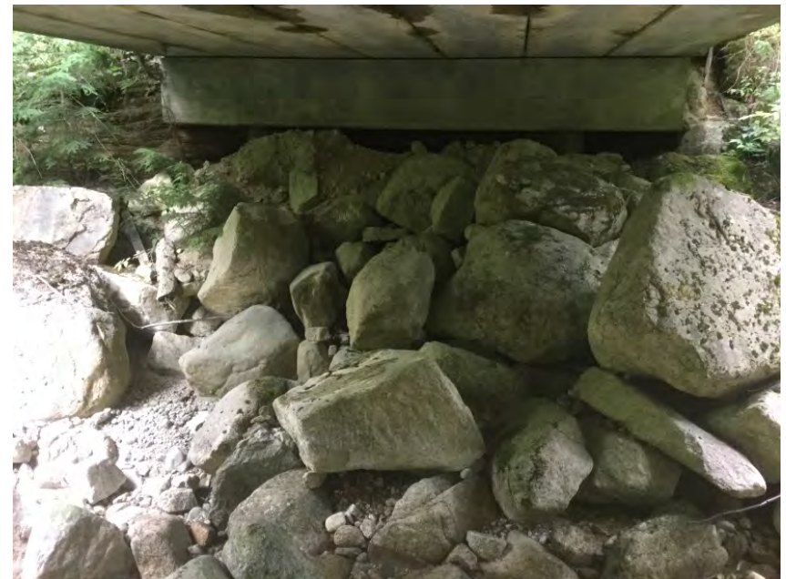
Right Bank Abutment when facing downstream
