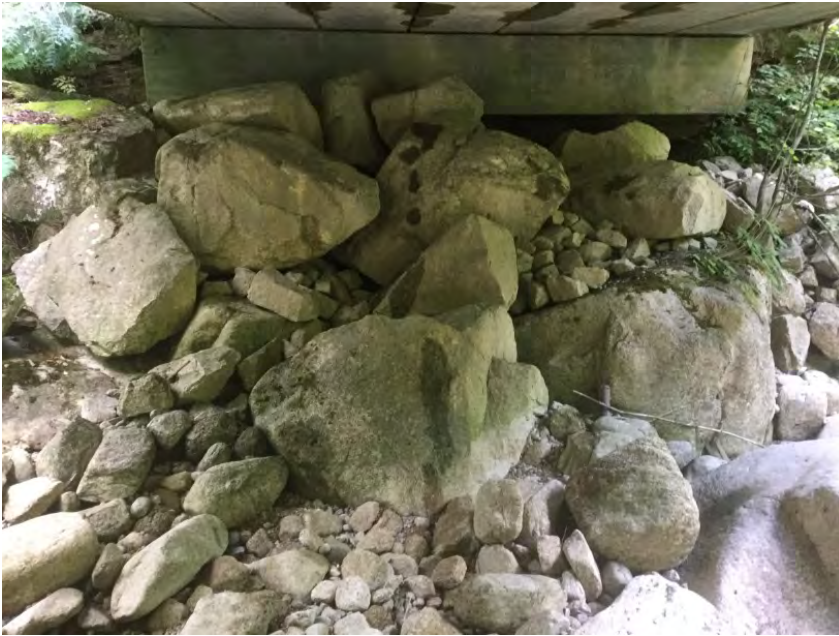
Left Bank Abutment when facing downstream
