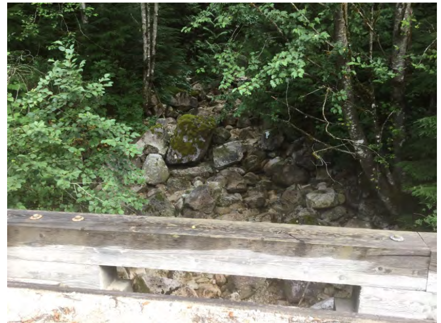
Looking upstream from deck
